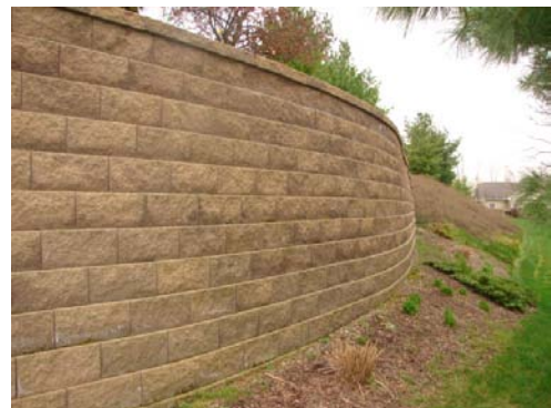
The long and high retaining wall installed in 2011 in good condition.
