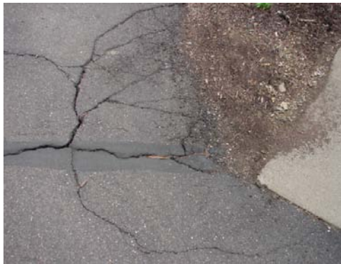
Asphalt cracking along edges of the driveway.
