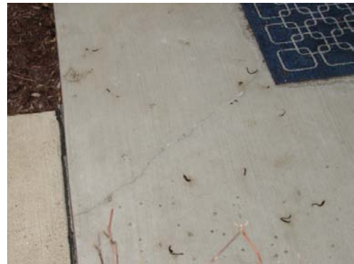
Minor crack in unit leadwalk.
