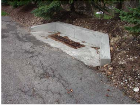
New drain with concrete curbing. New asphalt mill and overlay will need to slope accordingly.
