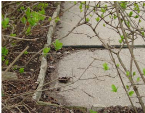
Leadwalk section has settled, causing a tripping hazard.
