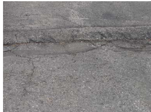
An asphalt curbing across common driveway to control drainage This condition needs to be corrected when asphalt is milled and overlaid.
