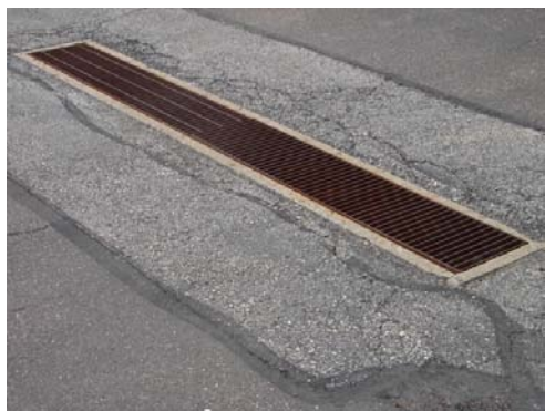
Typical storm drain at some driveways in front of garage door
