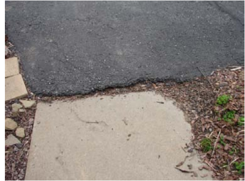
New asphalt overlay causes tripping hazard.
