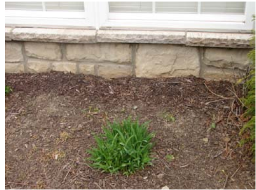
The stone veneer has some deterioration where covered by mulch. Remove mulch.
