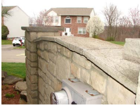
The rear of stone monument with cut stone cap. This stone area as well as other areas will eventually need tuckpointing/repair.
