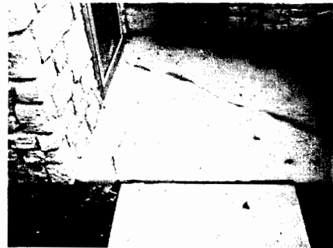
Stoop cracking
