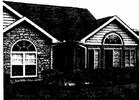
Typical unit roofline
