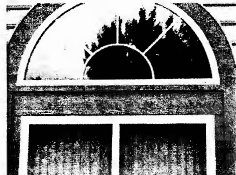
Typical painted synthetic wood window trim
